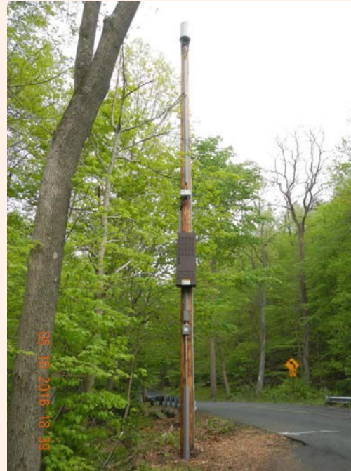
Installation on New Verizon Telephone pole or Existing Verizon Telephone/PSE&G/ACE pole
