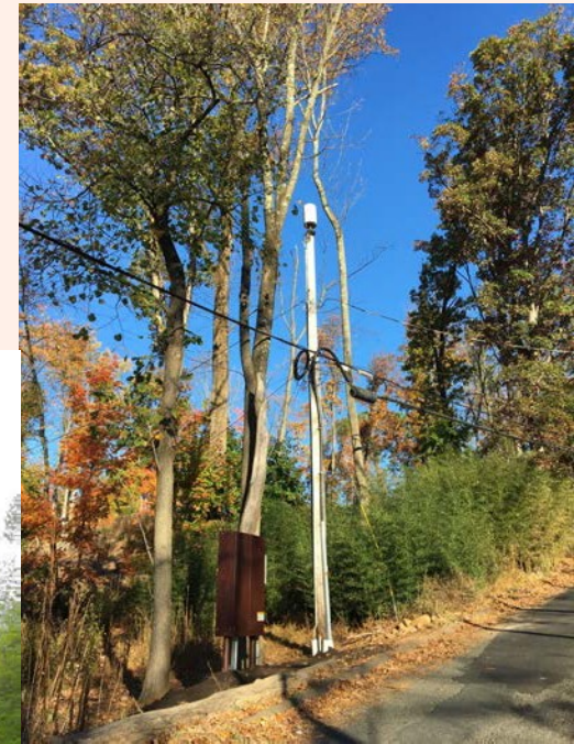
Installation on Existing JCP&L Pole
